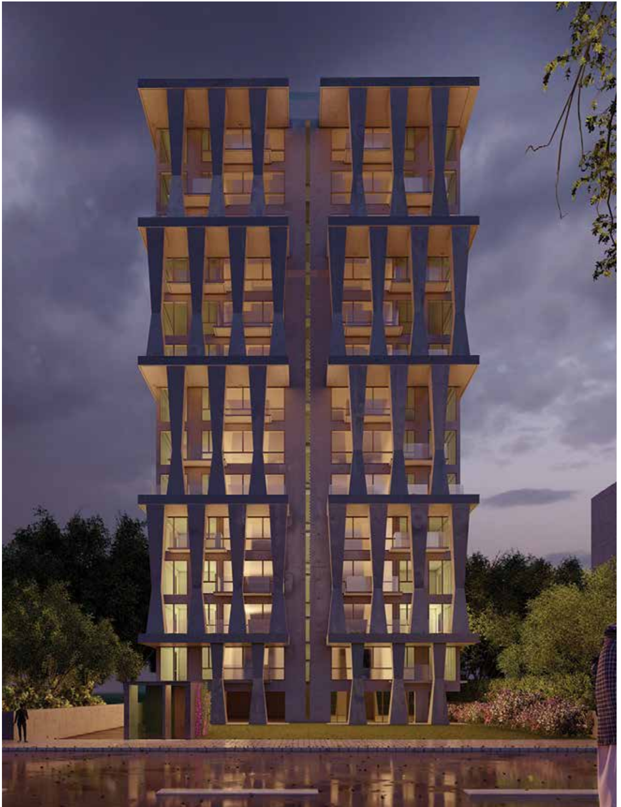
"The Crest" Plot # 10, Road # 3, Dhanmondi, Dhaka
