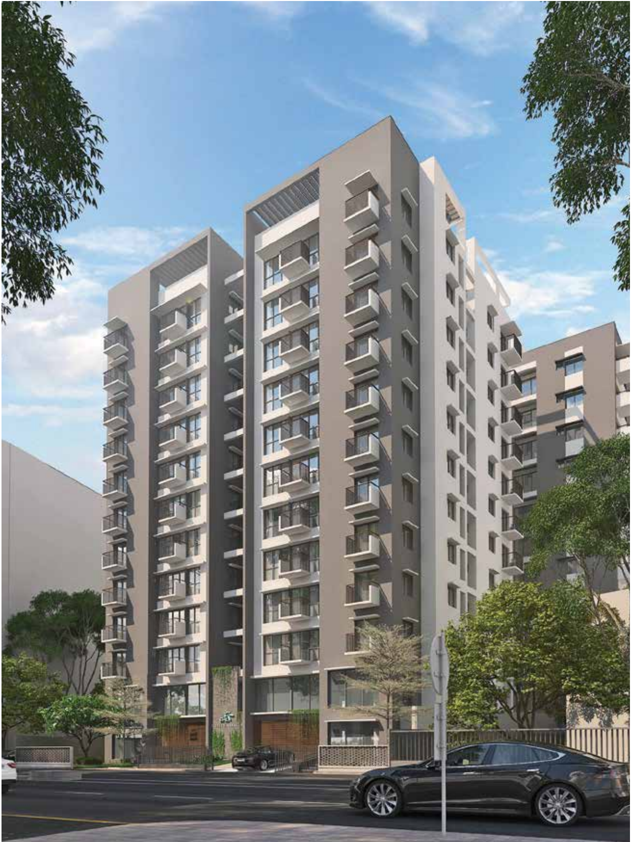
"Eastern Nabarun Residences" Plot # I/1- ka, Avenue # 4, Section # 2, Mirpur, Dhaka.
