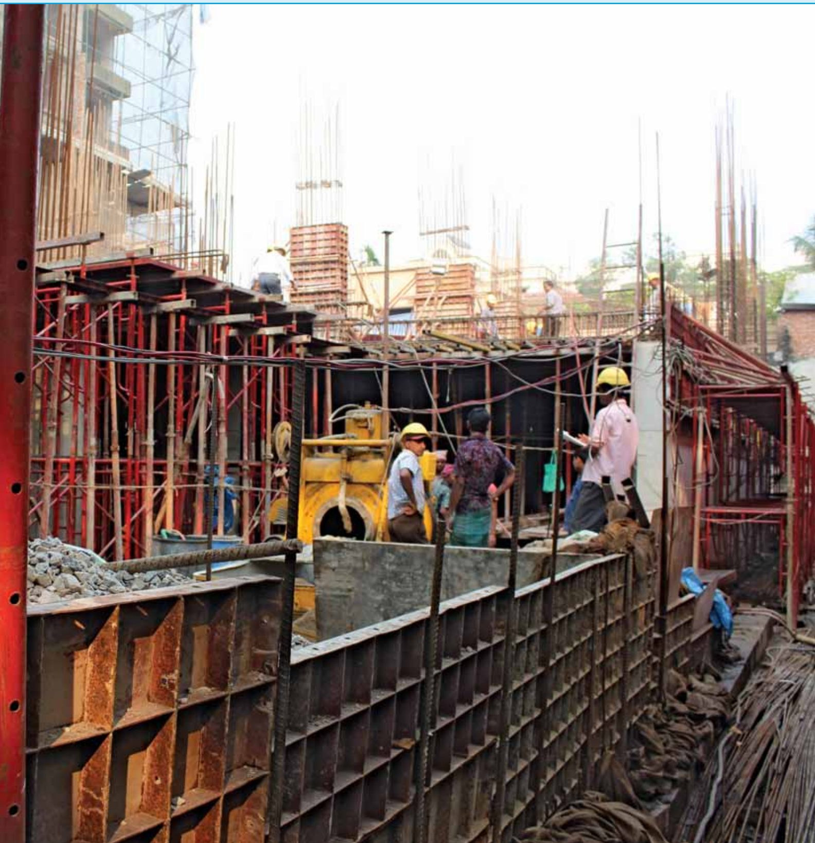
A view of the work
