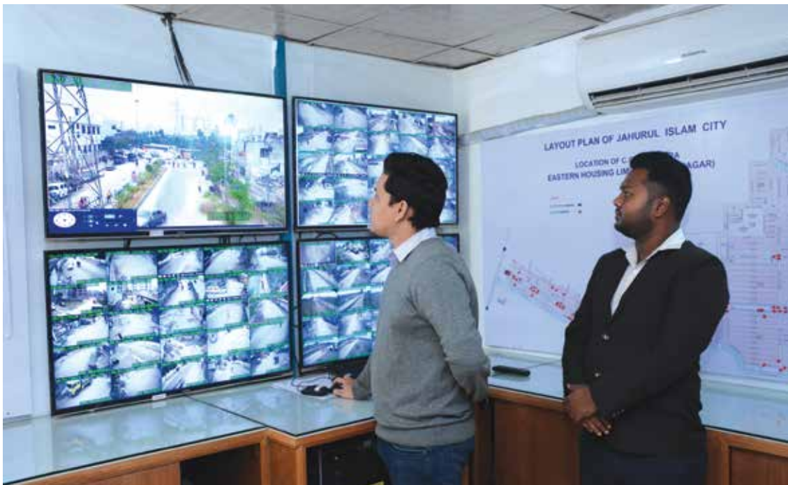
CCTV Control Room
